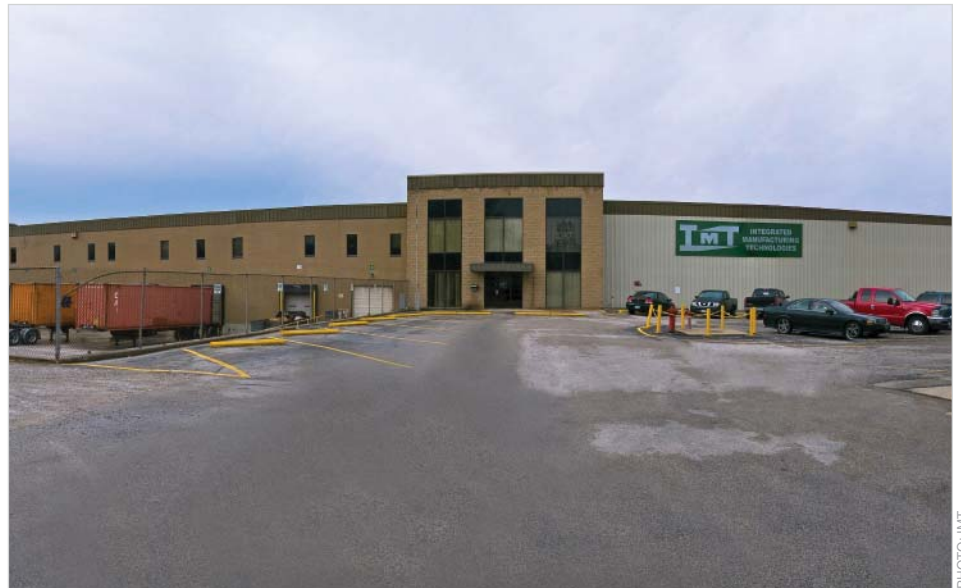
Integrated Manufacturing Technologies consists of 236,000 square feet and is located in Red Bud, Ill.
